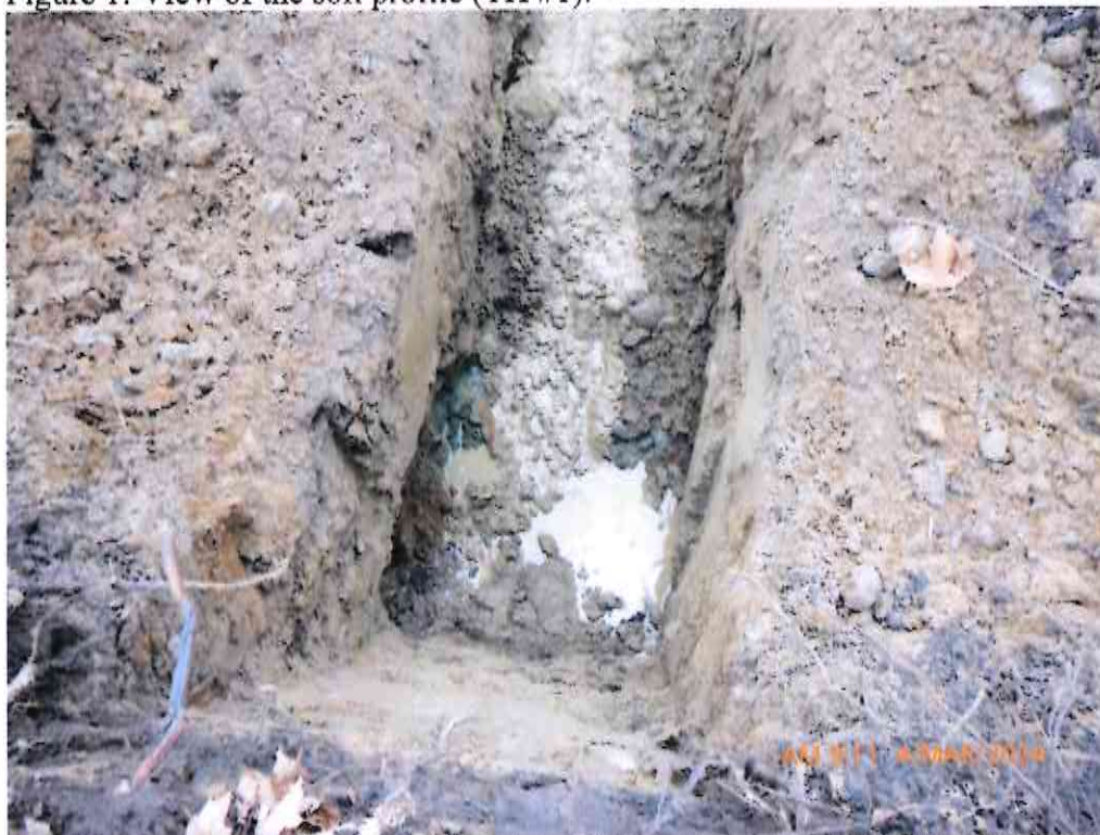
Figure 2: View of groundwater at 5.0 feet (60-inches) deep (TH #1).
